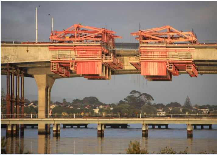
The Meeting Point: The north and south sections of the bridge are prepared to be joined together
