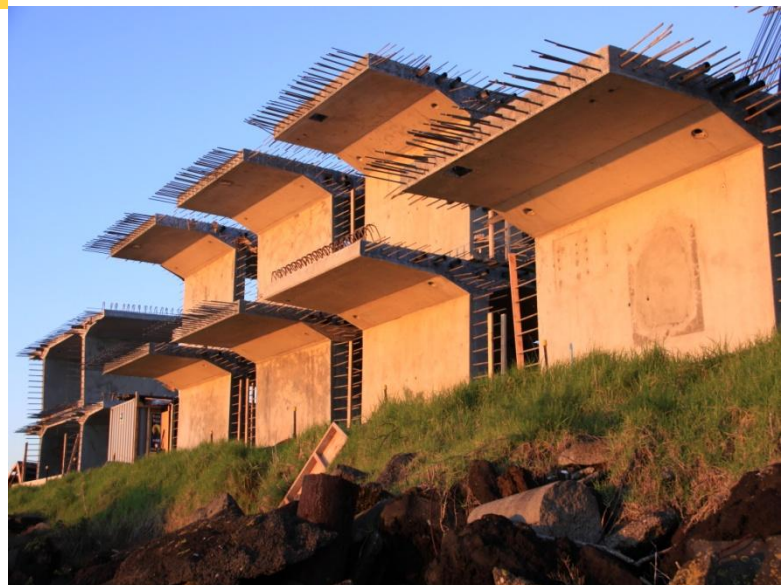
Pre-fabricated sections – a key innovation at MHX
